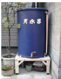
Fig.13 Rainwater harvesting tank 10
