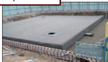
Fig. 14. Rainwater harvesting underground tank 9
